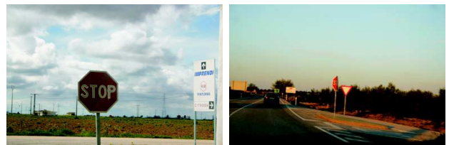
Fig. 7. Images from category "Deteriorated signs"
